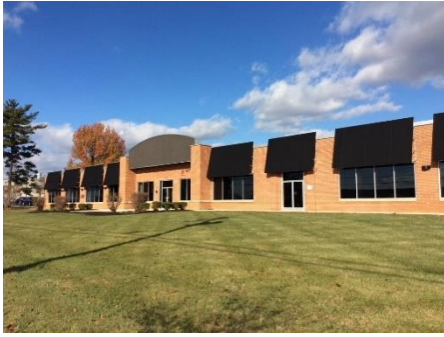
Front of Building
