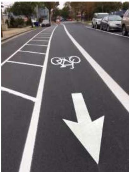
On northbound North Market, the new 5-foot wide bike lane is separated from the parking lane with a marked 5-foot wide buffer. Soon, green paint will be used to selectively mark sections of the bike lane, primarily at intersection transition areas, and a bicycle box at the signalized intersection with Ninth Street. The project retains on-street parking along both sides of the roadway and creates a defined northbound through travel lane to address previous traffic and bicycle safety concerns.
